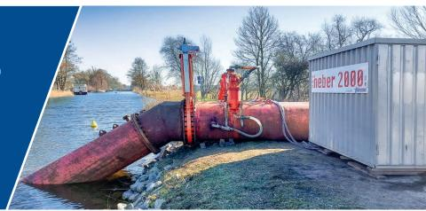
The heber 2000 uses the natural slope and its water level difference as an energy source and therefore does not require any external drive energy. External energy is only used for commissioning and maintaining operational readiness. Even in the event of a power failure, the system continues to pump for a longer period of time. This principle is therefore a particularly economical and reliable method of transferring large quantities of fluid.
