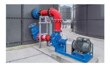
The Hidrostal screw centrifugal pump draws sludge from the source and returns it through a nozzle to provide optimum mixing energy and circulation of the tank contents.
